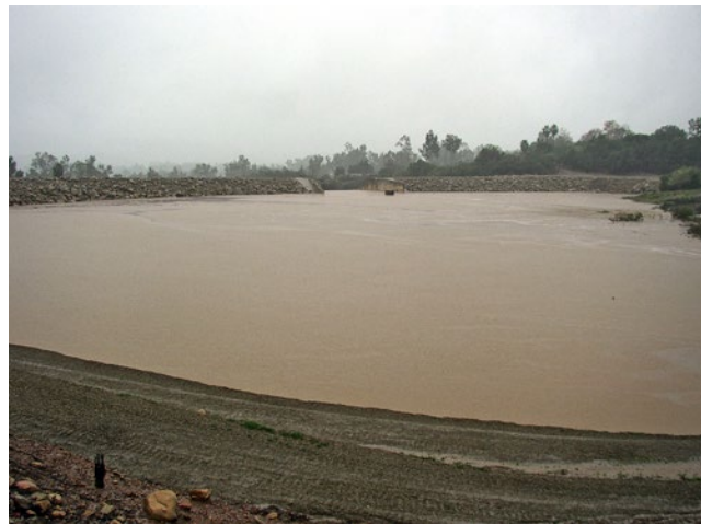
Stewart Debris Basin. Several debris basins at the base of foothills in the watershed trap sediment.
