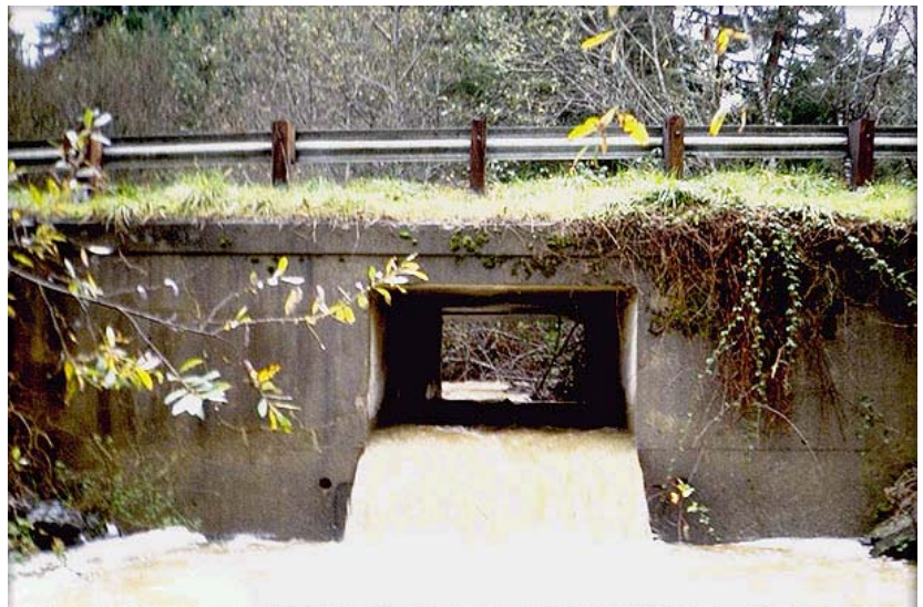
Figure 3. Leap Height and Low Water Depth Presenting a Potential Migration Barrier at a Box Culvert. Source: USDA Forest Service
