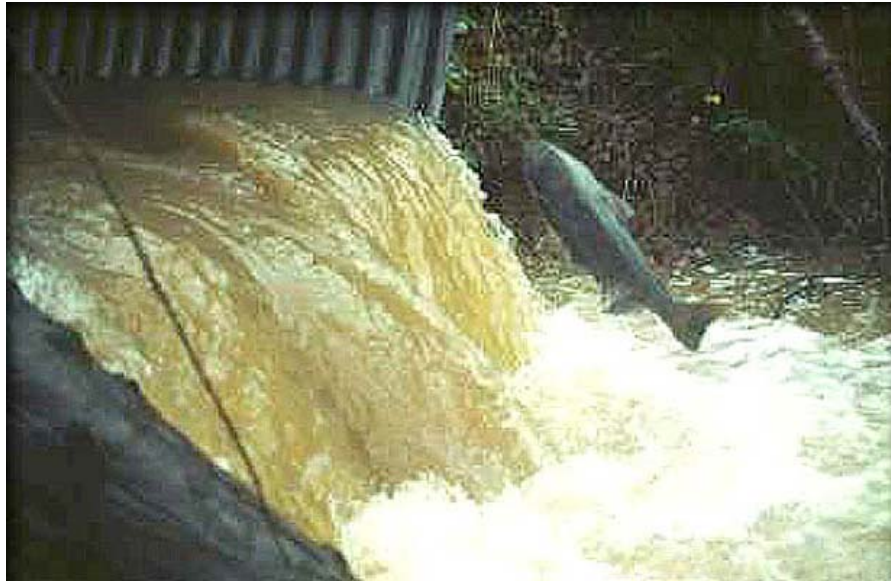
Figure 1. Adult Salmon Attempting to Enter a Culvert With a Leap Height Barrier. Source: USDA Forest Service.
