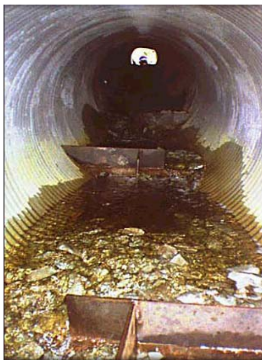
Figure 4. Baffles in a Modified Culvert Providing Velocity Refugia.
