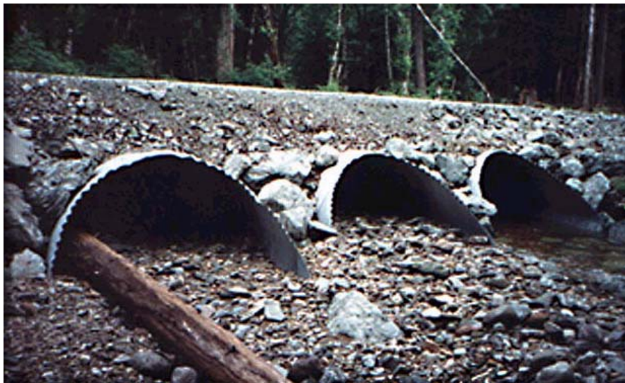
Figure 2. Passage Impaired by Sediment and Debris. Source: USDA Forest Service
