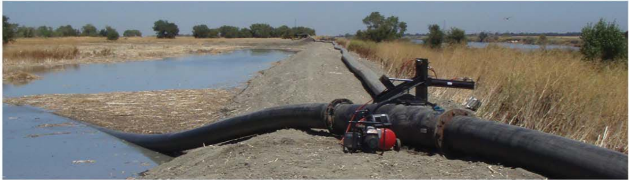
Figure 3. Photographs of Discharge Pipeline Y-valve
