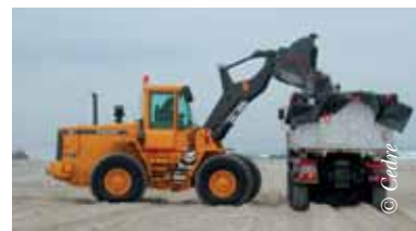
Truck and skip protected with plastic liner
