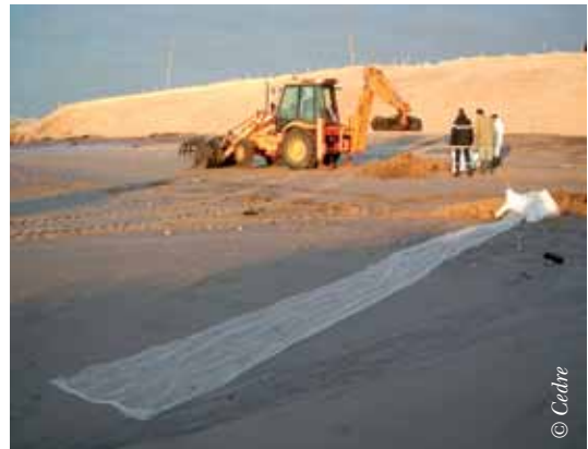
Implementation of netting to trap pollutant at high tide
