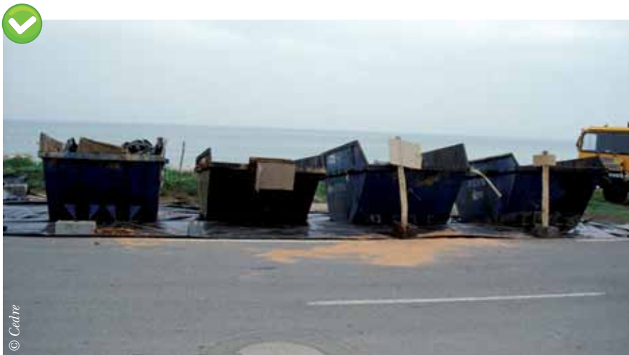
Skips for segregated waste storage
