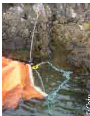
Cable attaching a boom to a rocky shore
