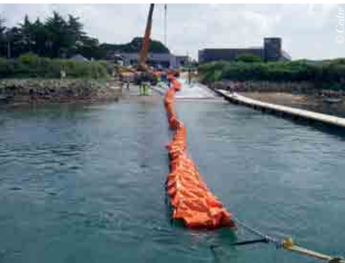
Deploying a non-compartmented foam-filled curtain boom
