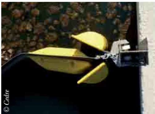
T-shaped slide rail with Teflon® bearings
