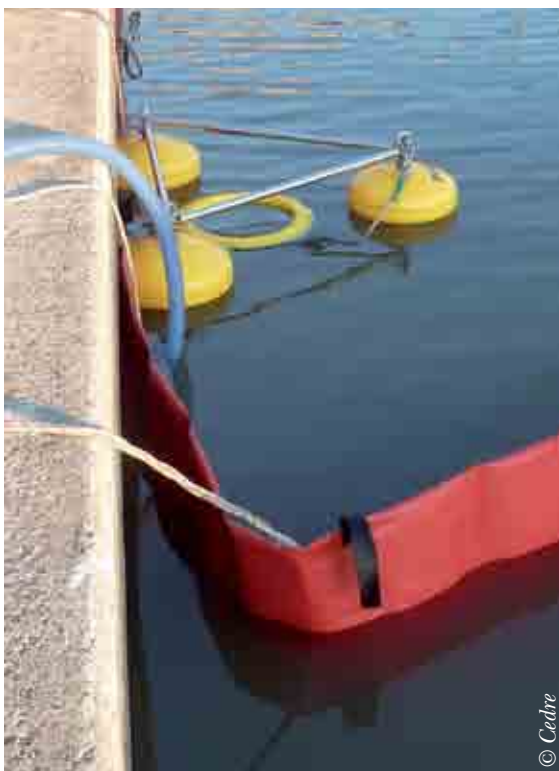
Ballasted rope to hold boom against dock wall
