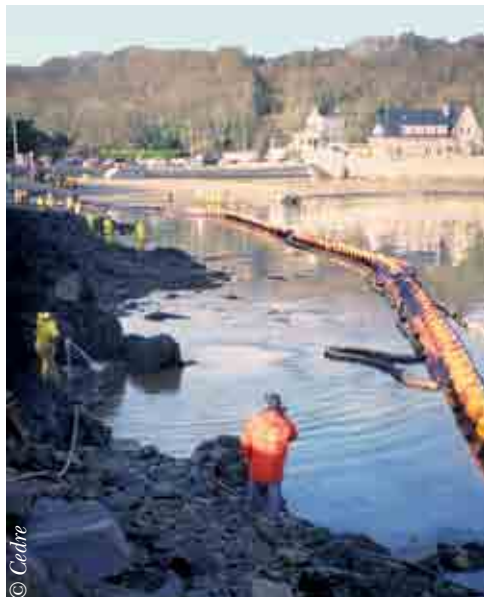
Effluent contained by booms at a riprap clean-up site
