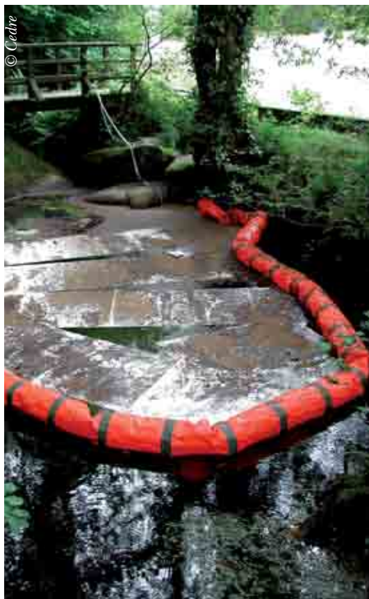
Containing and recovering oil using a boom and sorbents
