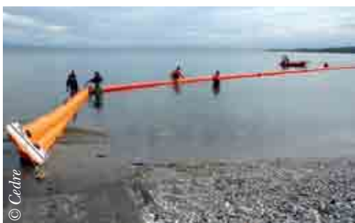
Deploying a shore-sealing boom from a slipway
