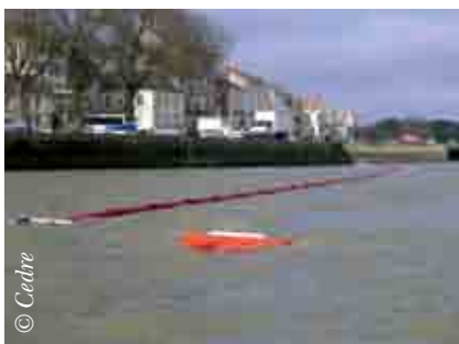
Setting up a deflection boom using a paravane
