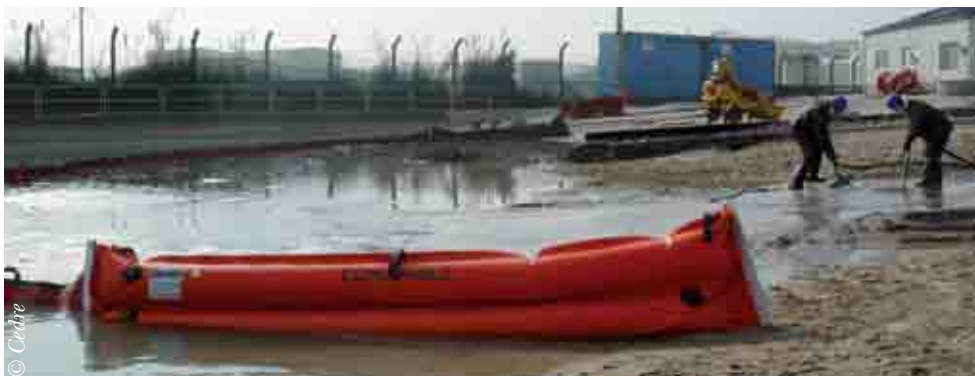
View of a clean-up site and a section of shore-sealing boom used to contain polluted effluent
