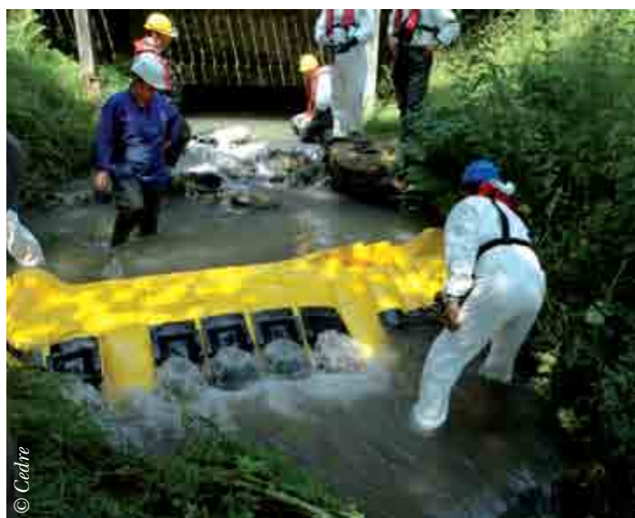
Deploying a flood protection boom
