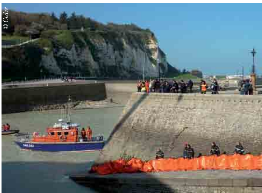
Deploying a non-compartmented foam-filled curtain boom
