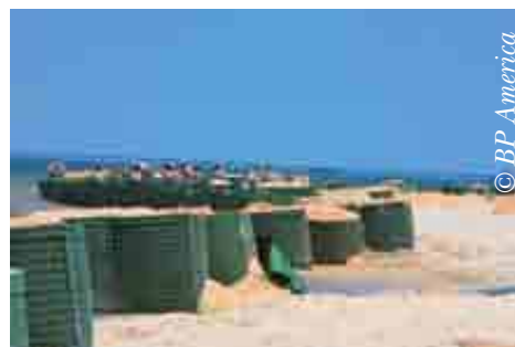
Constructing a protective dyke using sand-filled baskets, Deepwater Horizon, Louisiana 2010
