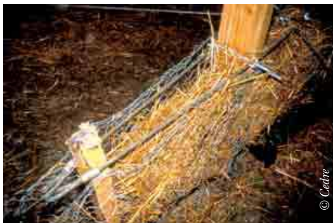
Protecting the sea inlet at Le Croisic, which feeds into Guérande salt marshes, using a straw filter barrier
