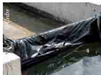
Run-off blocked in a concrete outfall using planks and plastic sheeting
