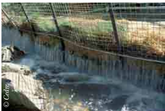
Example of alterations to a filter barrier to deal with increased current: replacement of piles with railway sleepers
