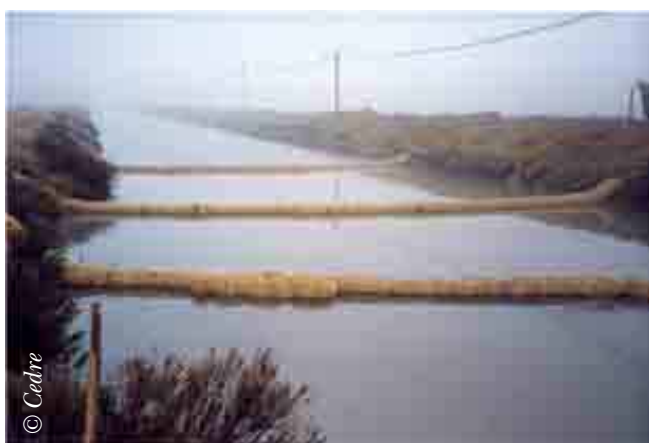
Protecting a stream in Bourgneuf Bay using straw-filled mussel nets
