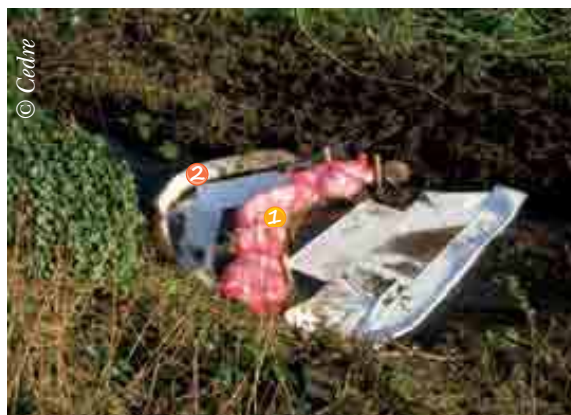
Reinforced measures: (1) filter barrier (double series of stakes with plastic mesh filled with sorbents) and sorbent pads and mats upstream (2) sorbent boom and pads
