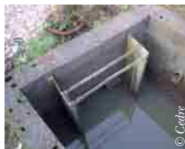
Track into which a perforated metal filter and sorbent fibres can be inserted
