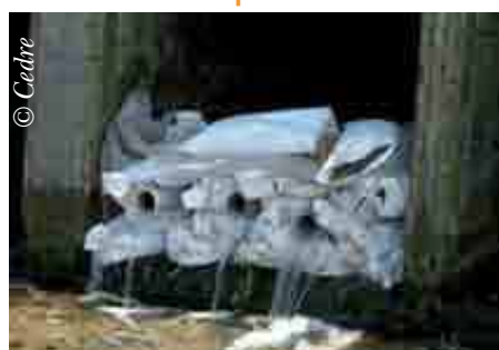
Barrier made using angled pipes and bags
