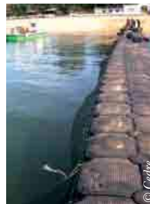
Protection by nets attached to a floating pontoon, Prestige spill, 2002
