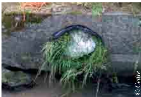
Plug made of geotextile, vegetation and plastic sheeting
