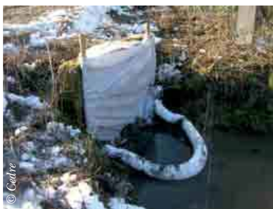
Filter barriers made of mesh, geotextile and straw together with sorbent booms
