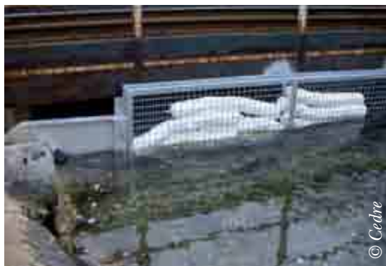
Retaining a spill at a discharge outlet using a filter cartridge
