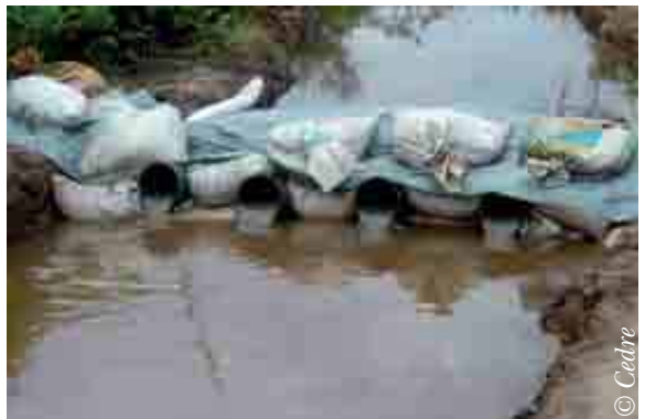
Barrier with angled pipes laid in an outfall (←) and in a stream (→)
