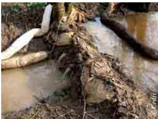
Earthen dam with angled pipes and sorbents
