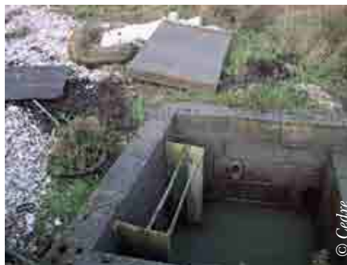
Filter cartridges made of perforated sheet metal and sorbent fibres installed in individual water intakes
