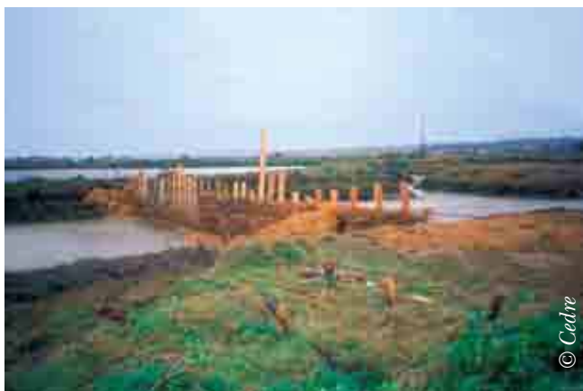
Protecting the sea inlet at Le Croisic, which feeds into Guérande salt marshes, using a straw filter barrier
