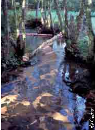
Straw barrier angled to hold strong in the flow of the river, Gironde 2001
