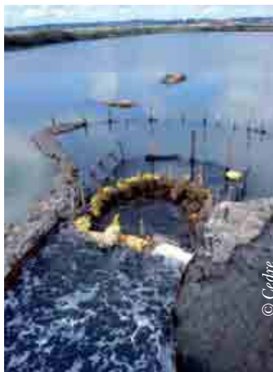
Filtration system made of oyster shells, feathers and pozzolana (porous volcanic rock) at the entrance to a mudflat
