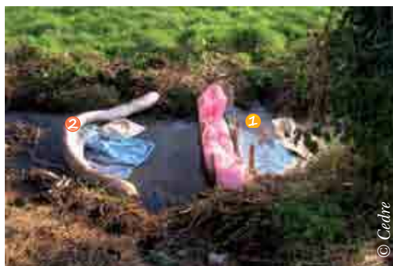
Reinforced measures: (1) filter barrier (double series of stakes with plastic mesh filled with sorbents) and sorbent pads and mats upstream (2) sorbent boom and pads
