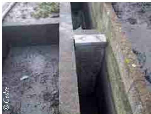
Filter cartridges made of perforated sheet metal and sorbent fibres installed in individual water intakes
