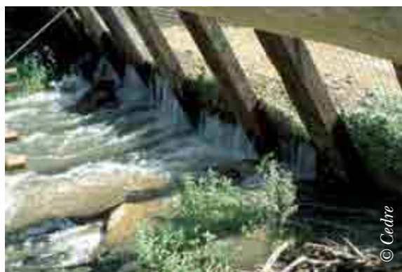
Example of alterations to a filter barrier to deal with increased current: replacement of piles with railway sleepers
