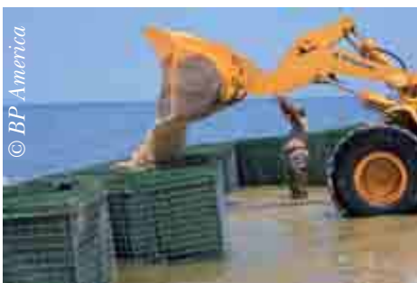
Constructing a protective dyke using sand-filled baskets, Deepwater Horizon, Louisiana 2010
