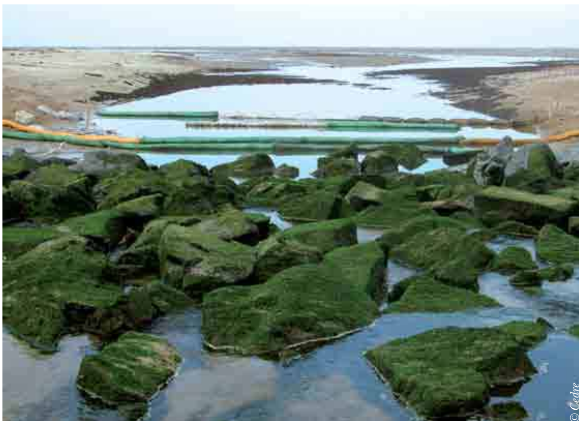
Sorbent booms and custom-made barriers at a river mouth at low tide, Manche 2009
