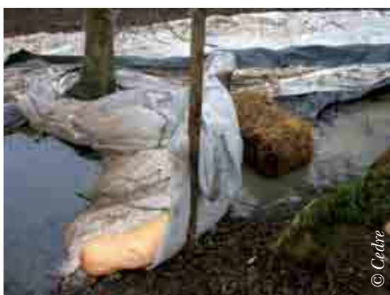
Filter barriers made of mesh, geotextile and straw together with sorbent booms
