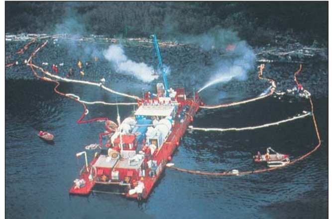
Hot water washing of a beach in Prince William Sound, Alaska, that had been oiled by the Exxon Valdez spill in 1989. Much of the shore life could not survive temperatures that reached 60°C.
