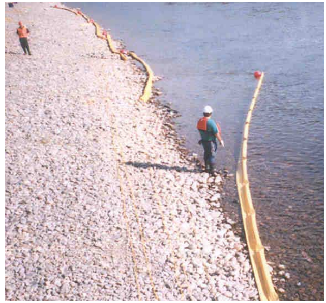
First boom is deployed.
