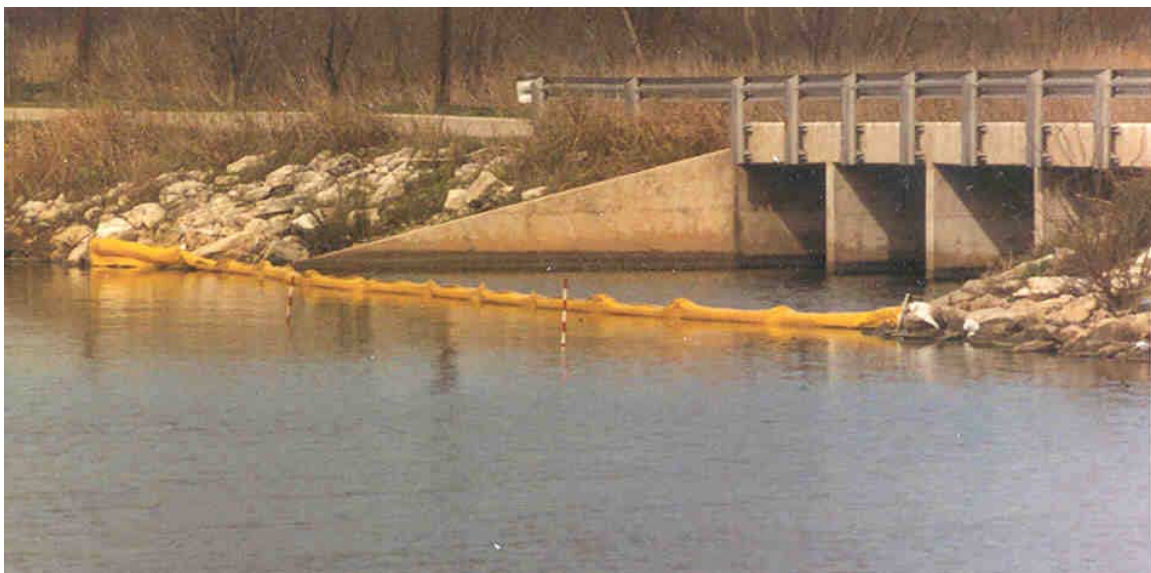
Figure 4-6. Exclusion booming of side stream.
