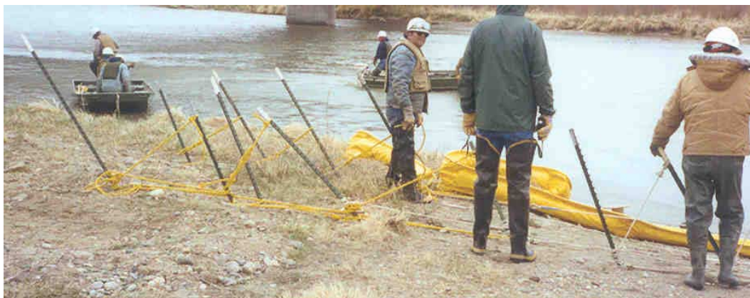
Figure 8-9. Multiple booms being anchored (DOWCAR, 1997).
