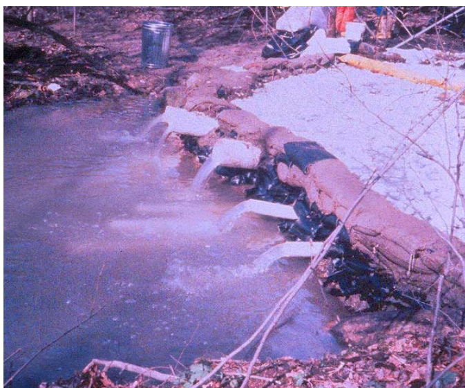
Figure 4-22. Sandbag underflow dam.
