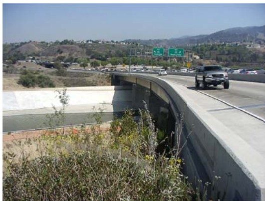
Urban Transportation and Flood Control
