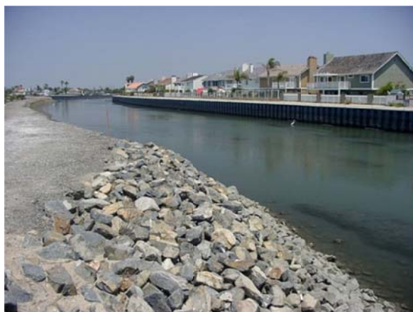
Wetland Fill - Santa Ana River Estuary
