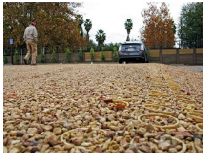
Pervious Parking Lot, Ojai Photo courtesy of Lisa Brenneis
