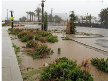
Bioswale, Surfers' Point, Ventura
