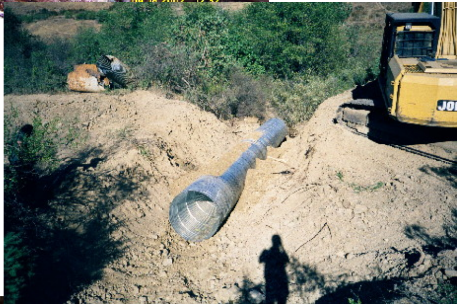
Stream Crossing Upgrading: Replacement of stream crossings deficient either in size or design.
