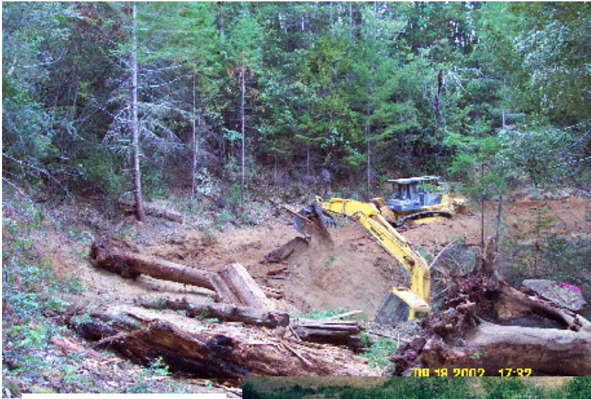
Road System Decommissioning: Obliteration and storm-proofing of dysfunctional or unneeded roads.
