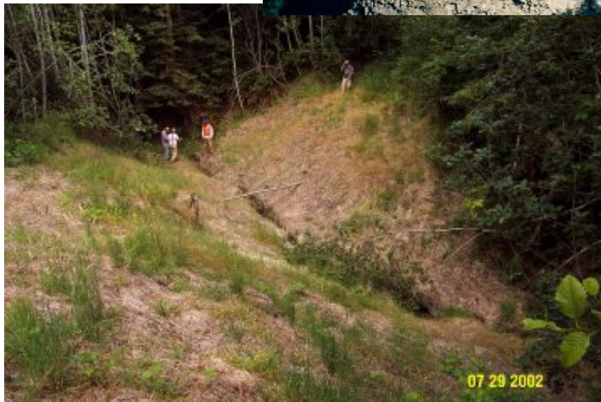
Stream Crossing Decommissioning: Removal and excavation of stream crossings to restore natural channel characteristics.
