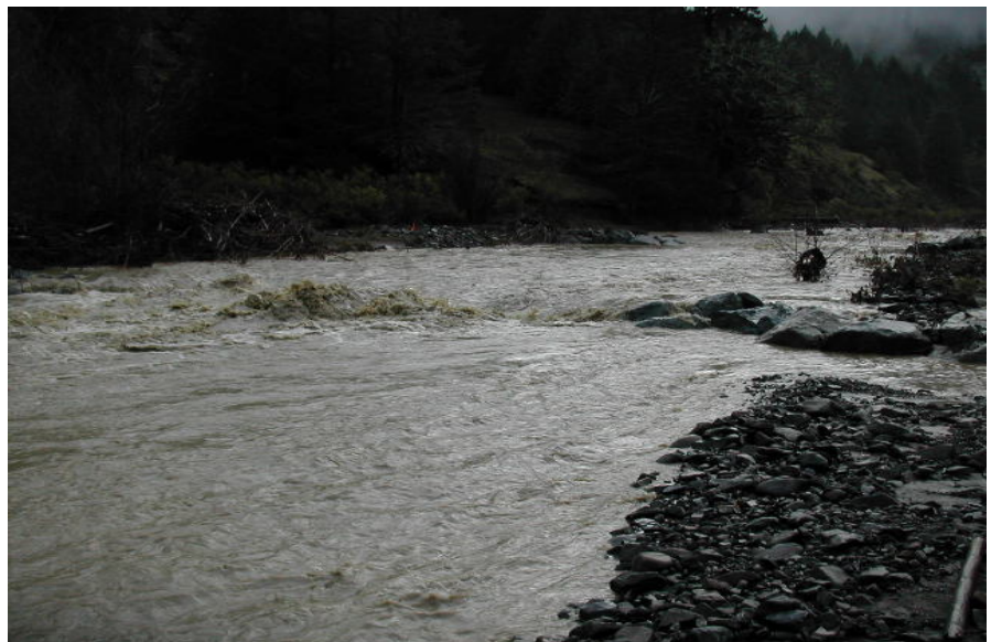
Figure 3. Instream Habitat Restoration Structure During Winter Flows. High flows going over boulder weir structures on December 23, 2002, at Bull Creek, CA.
