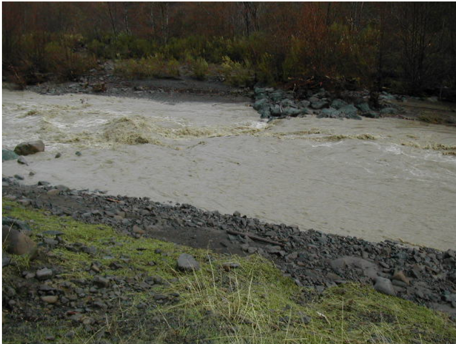
Figure 2. Photograph of Instream Structure at High Flow. Opportunistic photograph of boulder weir in Bull Creek during peak flow event (12/2002). Area of low velocity on right bank is visible, while a standing wave below the structure is evidence of hydraulic forces acting on the bed to scour out a pool. Photograph courtesy of Bill McDavitt.
