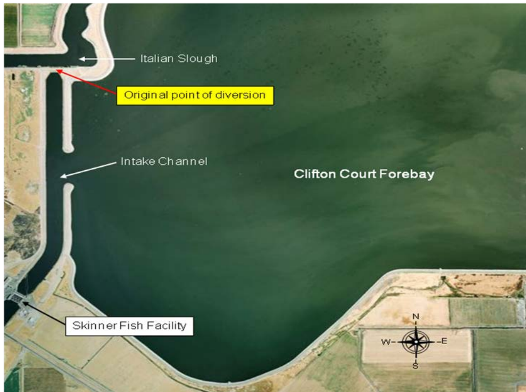
Figure 3. Aerial view of Clifton Court Forebay showing the intake channel leading to the SDFPF and the original diversion point for exporting water.
