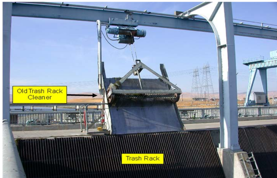
Figure 11. View of the old trash rack cleaner and old trash rack.
