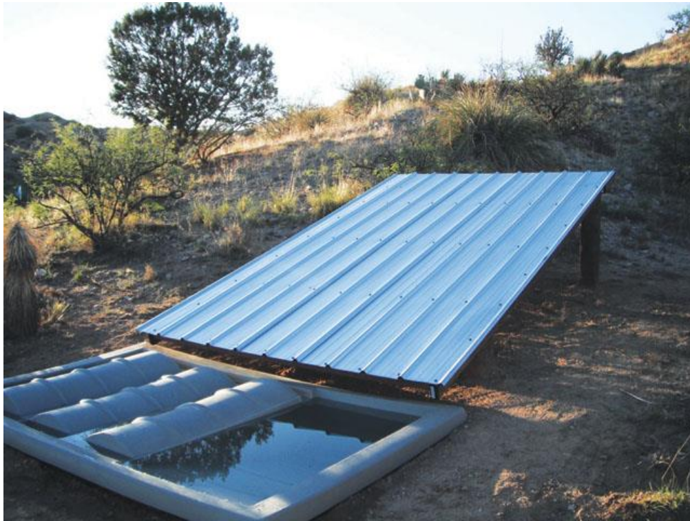
Figure 1. Shown here is a Rainmaker dome-top guzzler with the adjacent rainwater collection system.
