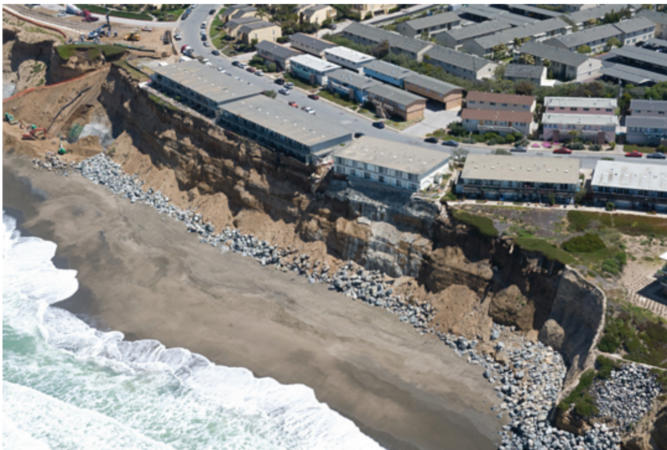
FIGURE 6.3 Erosion of poorly consolidated sedimentary cliffs at Pacifica, south of San Francisco, is threatening these apartments, and residents have had to move out. Riprap protection has been placed at the toe of the bluff in an attempt to slow the erosion. SOURCE: Hawkeye Photography.
