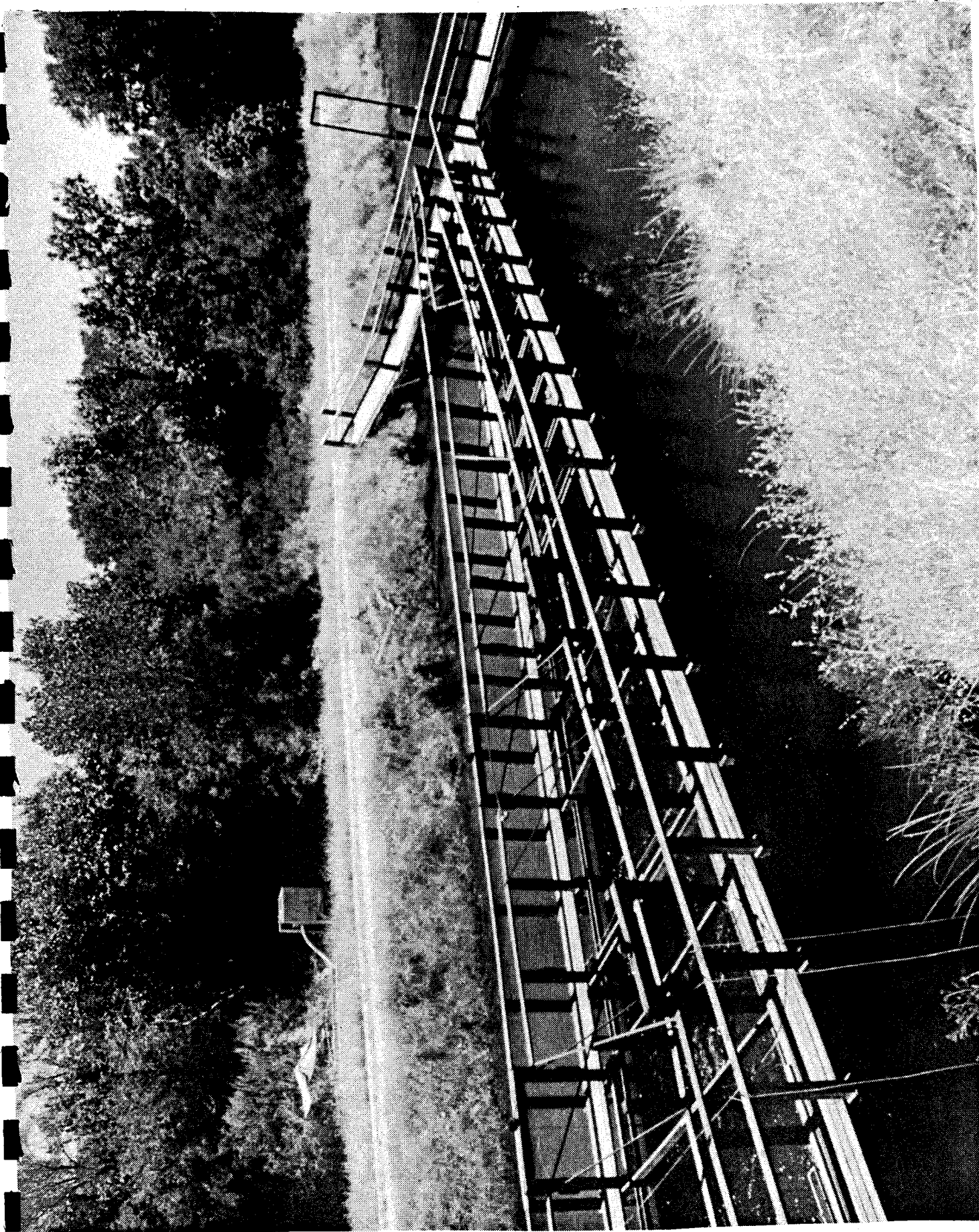
Figure 16. Hallwood-Cordua Irrigation diversion fish screen facility. The vertical wall V-screen is in the foreground, the flow control tower is visible in the upper left. View from the right bank of the diversion canal.
